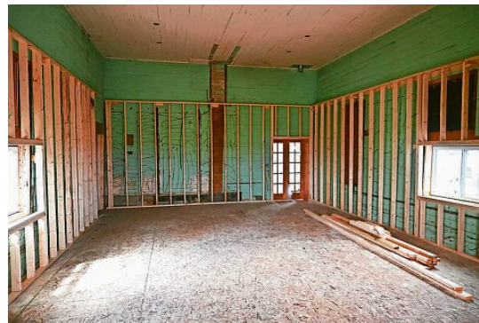
The old Algansee Township Hall at 378 S. Ray-Quincy Road was gutted ready for renovation into the new branch library. DON REID/COLDWATER REPORTER
